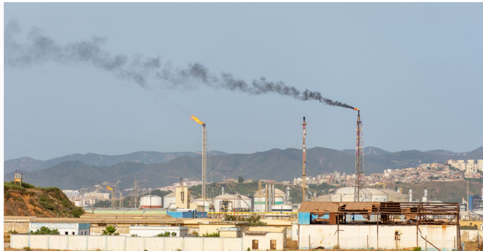
Sonatrach’s oil refinery in Skikda, Algeria. © hamdi bendali / Shutterstock
